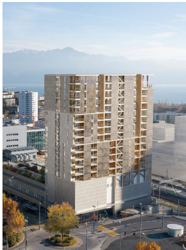
Malley Phare Source: Chantiers Magazine et CCHE
